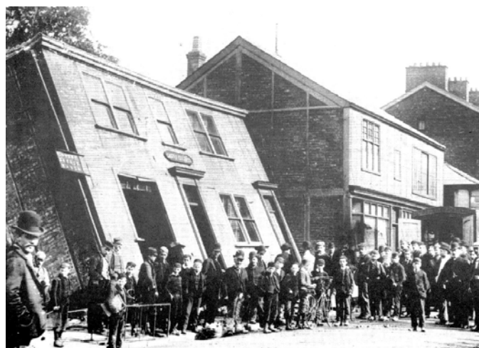
Figure 5: Damage at Castle street, Northwich, 1894, following “bastard brining”.
