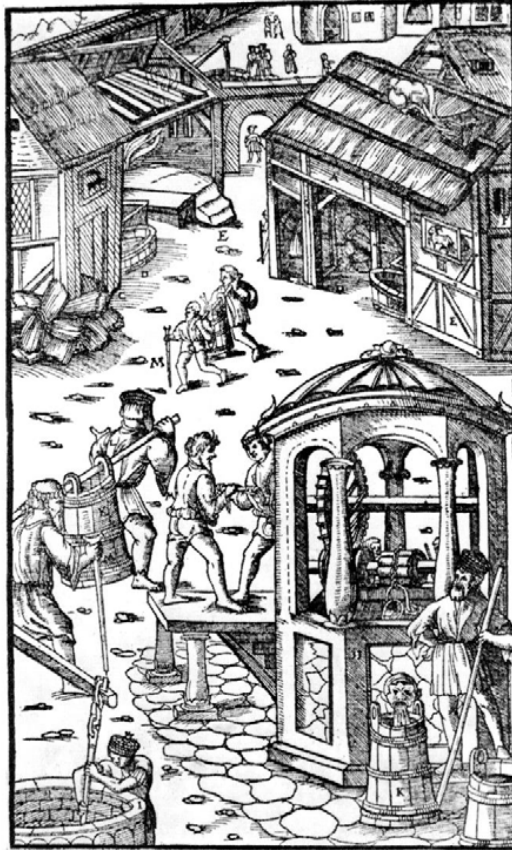
Figure 1: Manually operated bucket elevator brine pump. From Crotagino and Wilke (2014)
