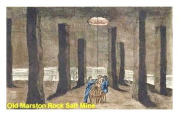
Figure 3. Painting of the Old Marston Rock salt mine in Cheshire, UK showing the very high extraction ratio and very thin pillars. From Crotogino and Wilke, 2014.
