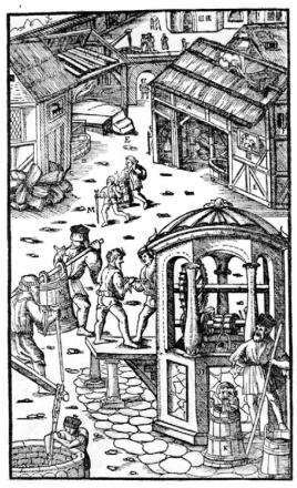
Figure 1: Manually operated bucket elevator brine pump. From Crotogino and Wilke (2014)
