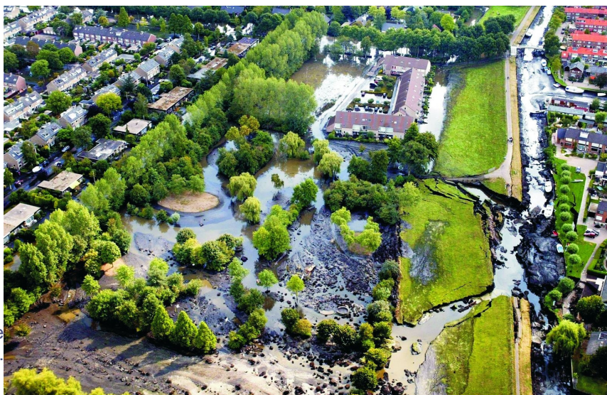
Figure 56: A breach in the Wilnis levee due to drought. Credit : STOWA.
