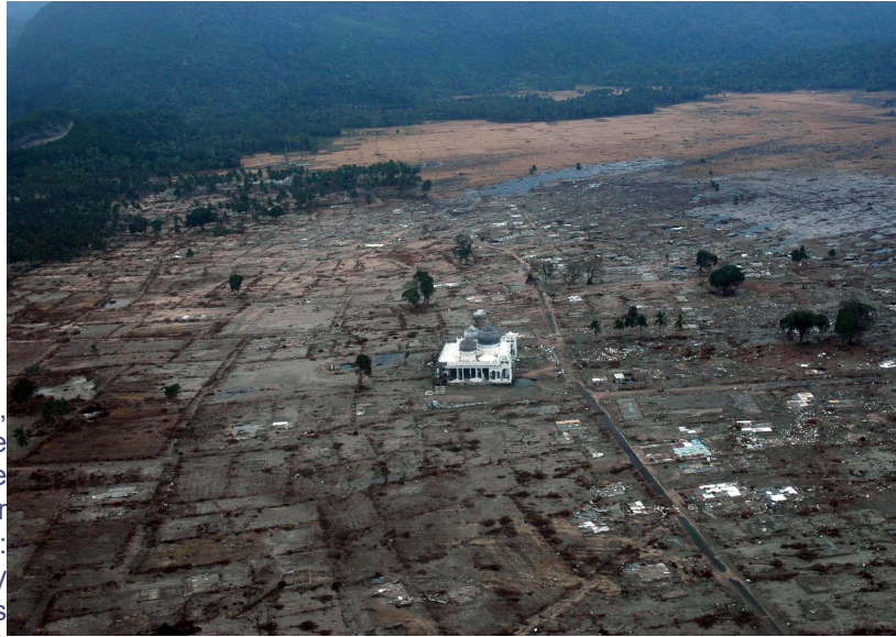
Figure 8: Aceh, Sumatra, Indonesia (Jan. 4, 2005). A lone mosque stands among the damage of a coastal village near Aceh, Sumatra, Indonesia. Credit: U.S. Navy photo by Photographer's Mate 3rd Class Jacob J. Kirk.
