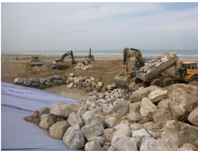
Figure 3. Construction site of Sangatte: implementation of armourstone on the levee (on the left) and of piles (on the right) - Source: DDTM 62
