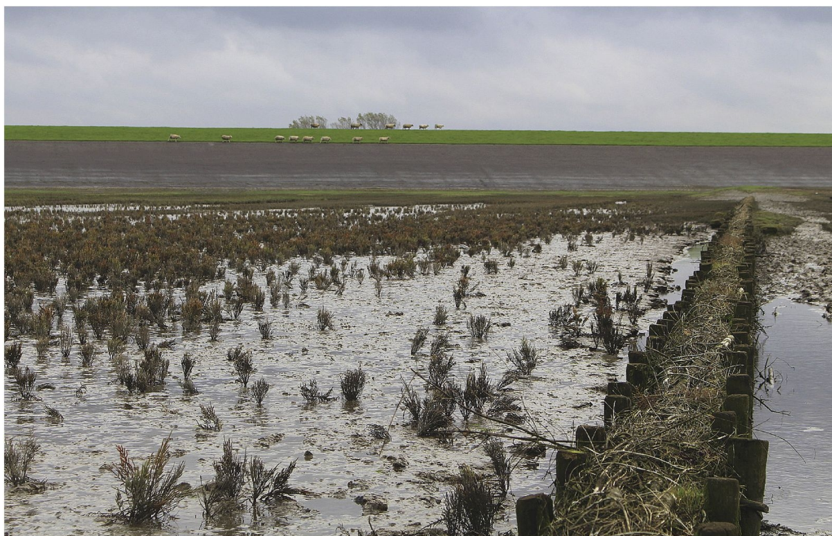
Figure 75: Brushwood dams in the Dutch Wadden Sea, which create artificial shelter for salt marsh vegetation from waves and currents. The levee is visible in the background. Credit: V. Vuik.
