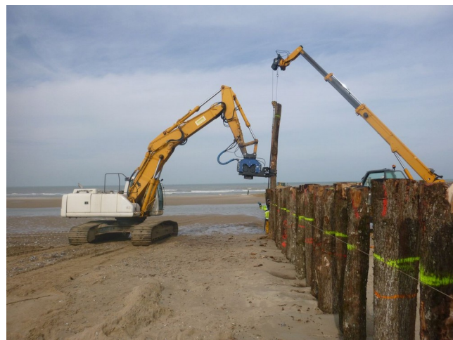
Figure 3. Construction site of Sangatte: implementation of armourstone on the levee (on the left) and of piles (on the right) - Source: DDTM 62
