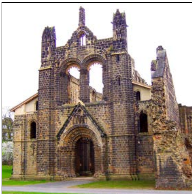
b – Kirkstall (West-Yorkshire, Angleterre). Abbaye cistercienne (c. 1156) Grandes baies jumelées contiguës de la tribune occidentale. © Tim Green-Flickr
