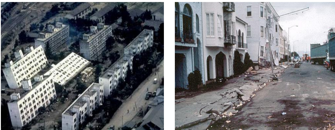
Figure 1.3 Damages caused by liquefaction events: Niigata Earthquake (Left) and Loma Earthquake(Right)
