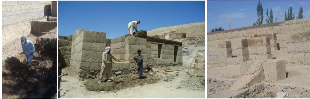
Figure 41: Preparation of loam and construction of pakhsa walls (photographs by the author)
