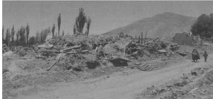
Figure 15: Typical damage in Nahrin district, walls collapsed completely, (Yeats and Madden, 2003)
