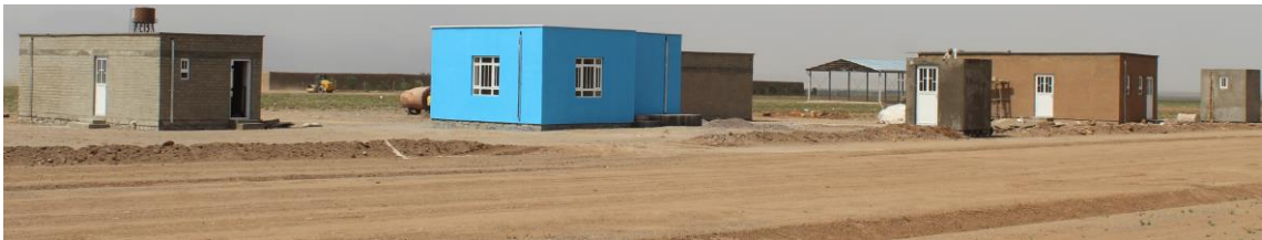
Figure 116: From left to right: units made with concrete block, interlocking block, and RE (UN-Habitat, 2017)
