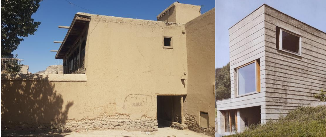
Figure 46: From left to right: traditional plaster in Kabul (Peacock House) and RE wall protected by ceramic support (Heringer, 2020)
