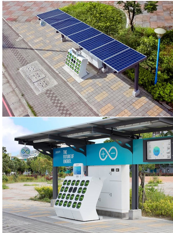
Figure 6.2: Gogoro’s solar-powered battery-swapping stations in Taiwan (Gogoro, 2017)
