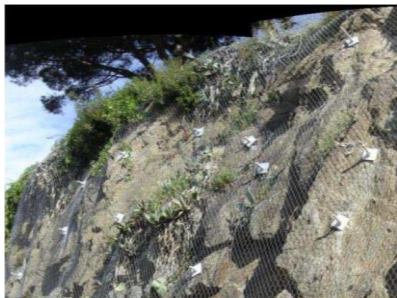
Figure 1-4 Tirants d'ancrage
