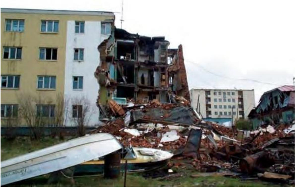
*Figure 33: Part of a building in the town of Chersky collapsed in June 2001 due to the weakening of the foundation built upon permafrost.*
