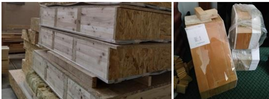
Figure 51. Prefabricated walls in production (Photo taken during the factory visit 2019, by Androšević)
