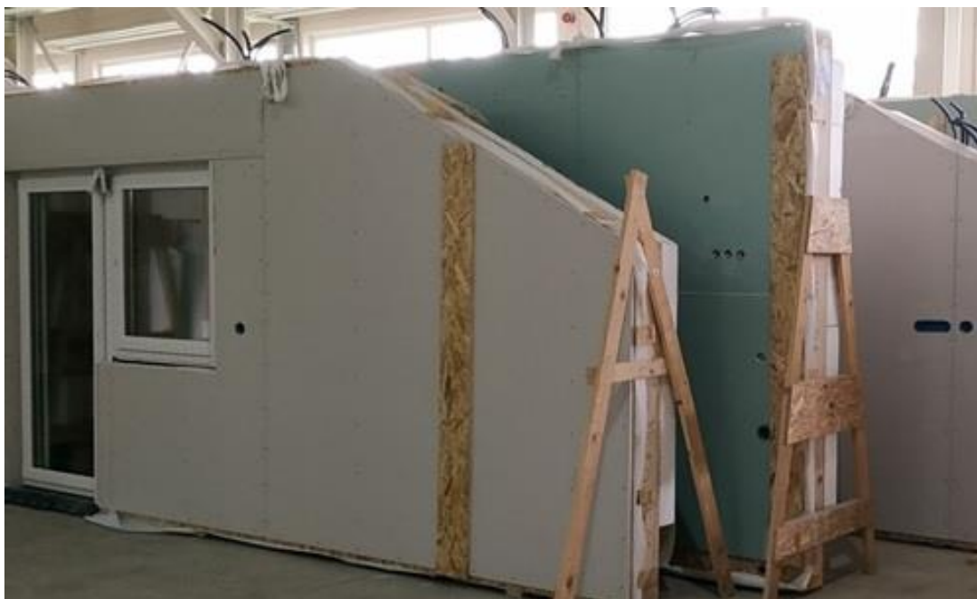
Figure 53. Prefabricated walls in the production (Photo taken during the factory visit 2019, by Androšević)
