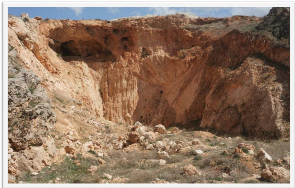
Figure L. 8. Another angle of the side of the quarry shows the impact on soils and vegetation. (Shaiban, IMBE).
