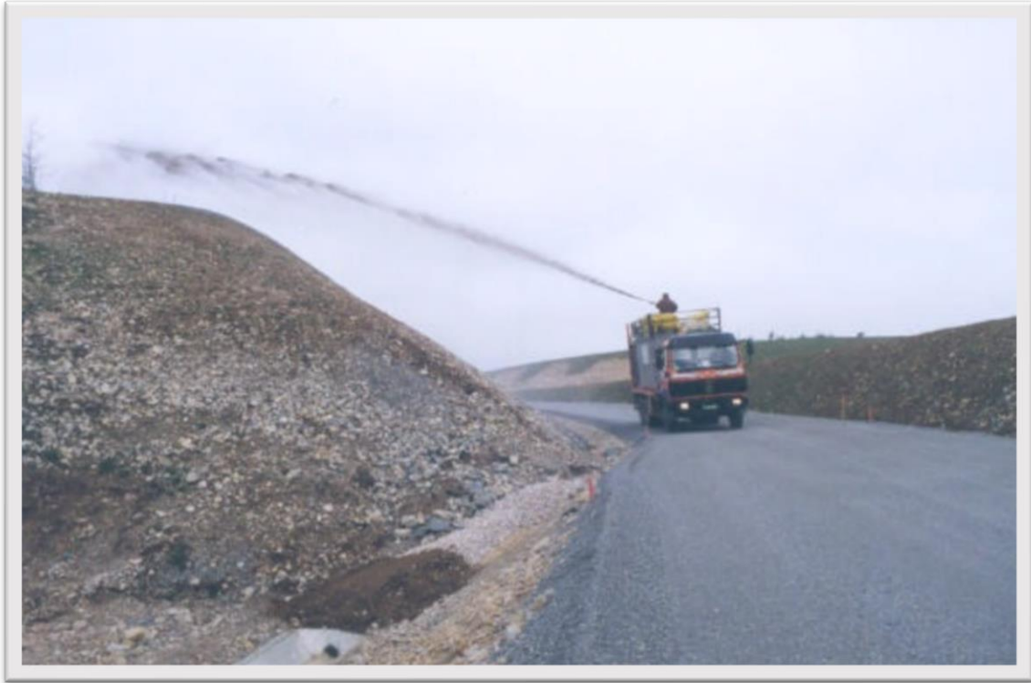
Figure 1. 1. Utilizing the hydroseeding technique as a restoration tool on a steep road cut slope
