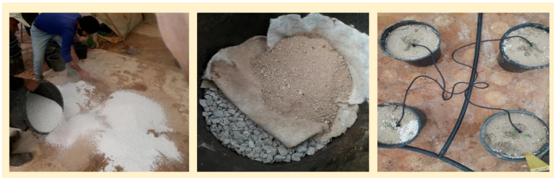
(a) Mixing perlite at a 10:1 ratio (b) Barrier amid pebbles & soil (c) Adding an irrigation system
