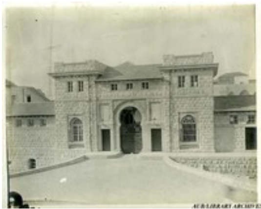
Figure 12 - Porte principale du SPC, Main Gate, fermée, 1917
