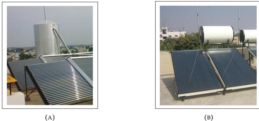
FIGURE 3.1: (a) Storage tank placed separately from the collector. (b) Storage tank placed on-top of the collector.
