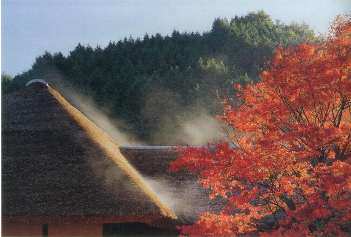
Figure 46 : Rosée de matin « As moisture accumulated in the gaps between the thatch expands as the sun rises, it evaporates and mist rises. » Takenaka, Asago, Hyogo (Japon), 1988 (« Harimayabonten Ikuno Head Shop », 2019, p. 174)
