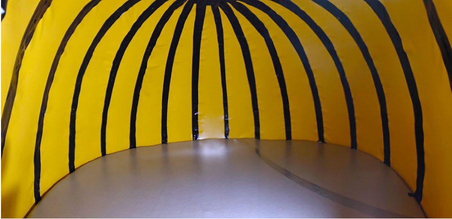
Figure 7.9: Inside of the inflated dome upon completion.
