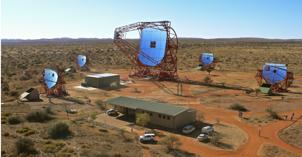
Figure 2.5: The H.E.S.S. array of IACTs. The phase one small telescopes CT1-4 are visible at the corners of the array. The large phase two telescope CT5 is at the center. Figure extracted from Ref. [138].
