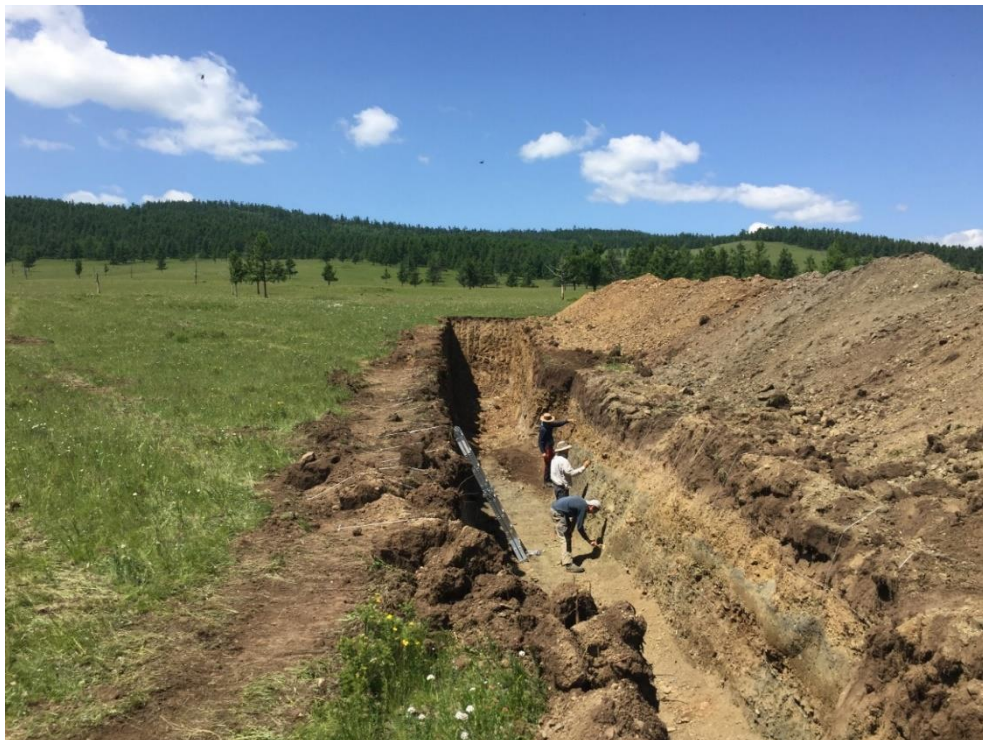
Figure 73. Field picture of trench 1 (T1); researchers are cleaning and brushing the trench walls before photographing, logging and sampling (photo by D. Battogtokh, July 2019).
