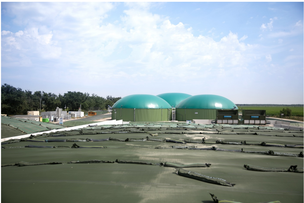
Figure 4: Pot-au-Pin biogas plant – view from a covered silage pit (@Constant Formé-Bécherat)
