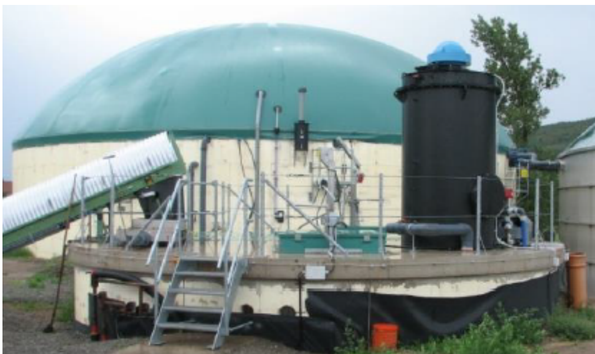
Figure 20: Picture of a semi-aerobic hydrolysis tank – from (Bionova-Biogas GmbH, website)
