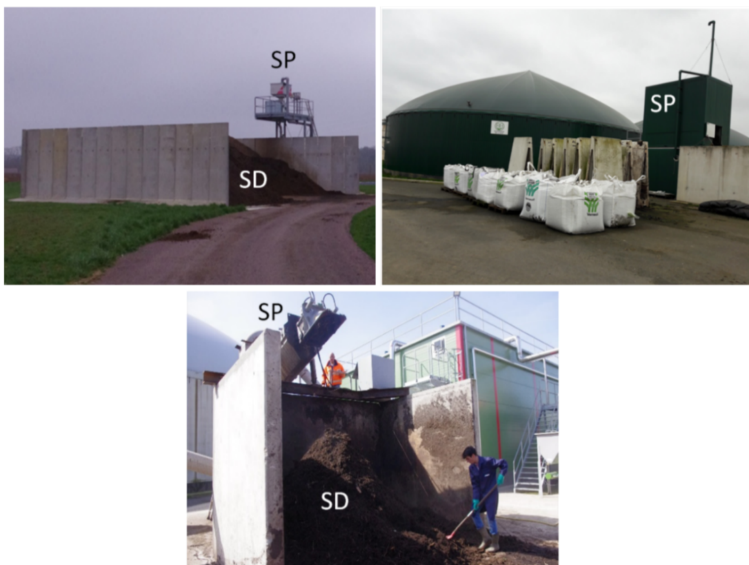
Figure 22: Examples of solid digestate (SD) sampling location. SP states for Screw Press
