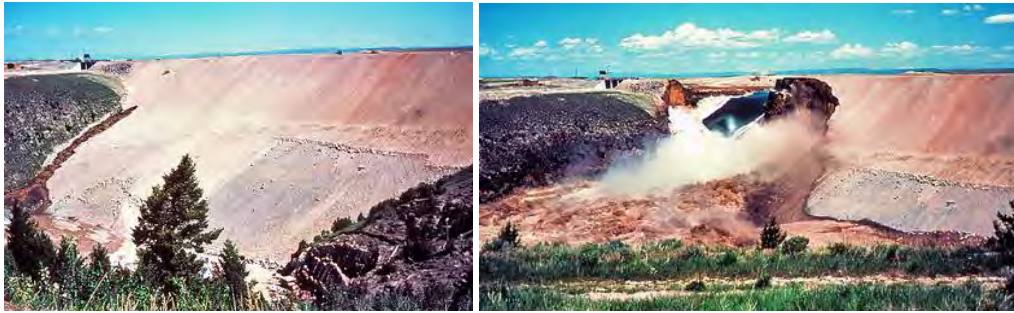
(a) Leak has started
