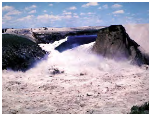
(c) Dam has collapsed
