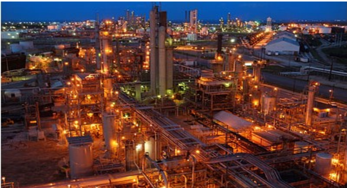
Figure 3-1: Typical industrial geometry (Petroleum Company LP refinery at Texas City, Texas)
