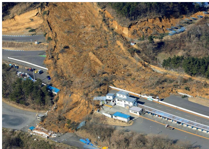
Figure 1.1: A landslide covers a circuit course in Nihonmatsu city, Fukushima prefecture, northeastern Japan, Sunday, Feb. 14, 2021. The strong earthquake shook the quake-prone areas of Fukushima and Miyagi prefectures late Saturday, setting off landslides and causing power blackouts for thousands of people. [Hironori Asakawa/Kyodo News]
