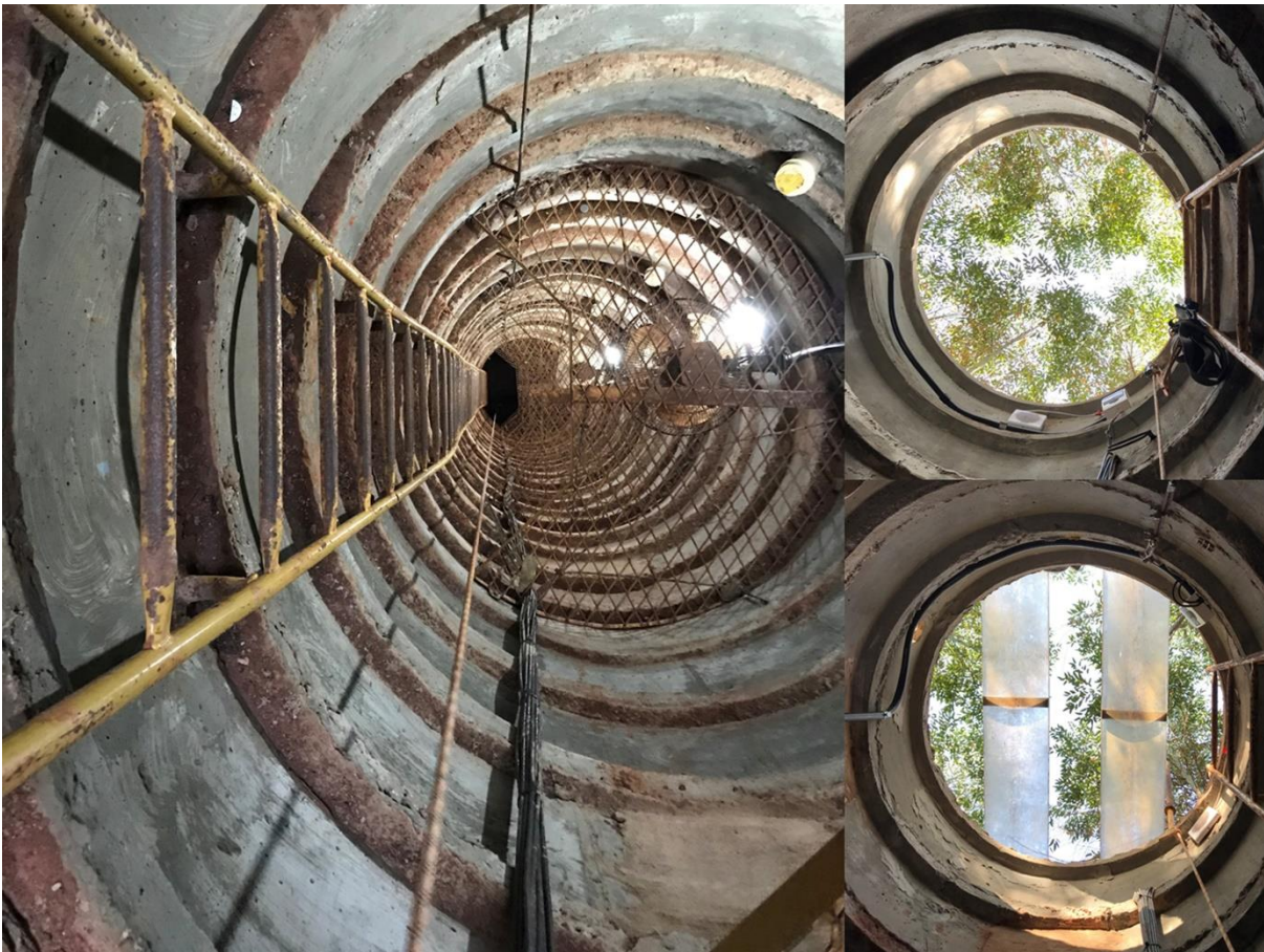
Figure III. 2: Deep permanent pit down to a depth of 17 m in throughfall exclusion experiment at the Itatinga Forest Science Experimental Station in São Paulo state.
