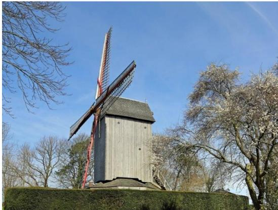
Figure 12. The Cassel (North) "pivot" type mill (Photo by PAT 2013, [www.moulins-a-vent.net](http://www.moulins-a-vent.net))
