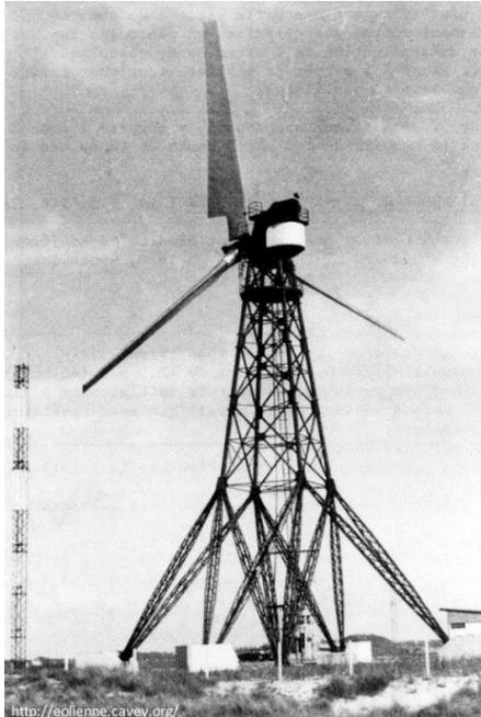
Figure 18. Machine of 35 m, 1 000 kW, Neyrpic wind turbines of Saint-Rémy-des-Landes. (Source: <http://eolienne.cavey.org/>)
