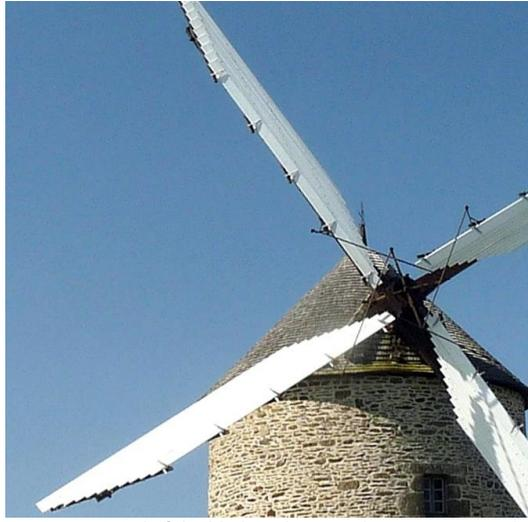
Figure 11. Detail of the blades whose angle can vary according to the wind speed. ( D. Serero)
