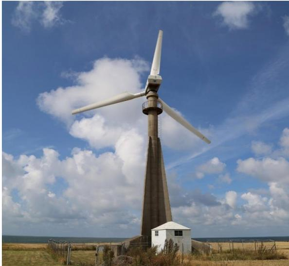
Figure 20. Gedser turbine in Denmark, on a reinforced concrete mast the origin of today's wind turbines (source: <https://fr.wind-turbine-models.com/>)
