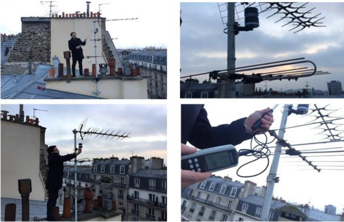
Figure 91. Installation of the anemometer on the roof of the building 136 avenue Parmentier, Paris 11ème. A TV antenna was used to support the device.
