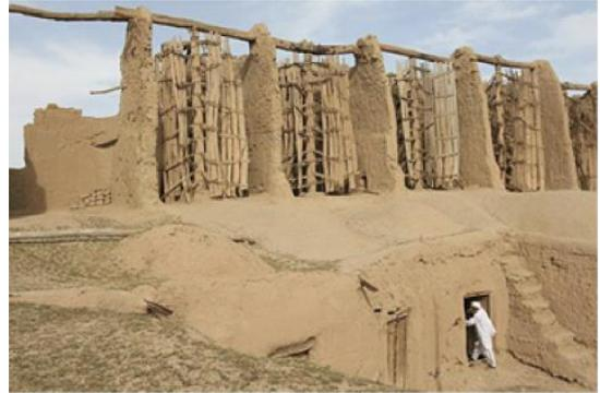
Figure 3. The vertical blades of the raw earth windmills partly go up against the wind and limit the speed of the device, src: National Geographic, photo Reza Azizfarkhani
