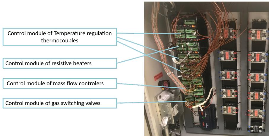
Figure 4.10: Picture of the electronic modules of the research-scale ALD system
