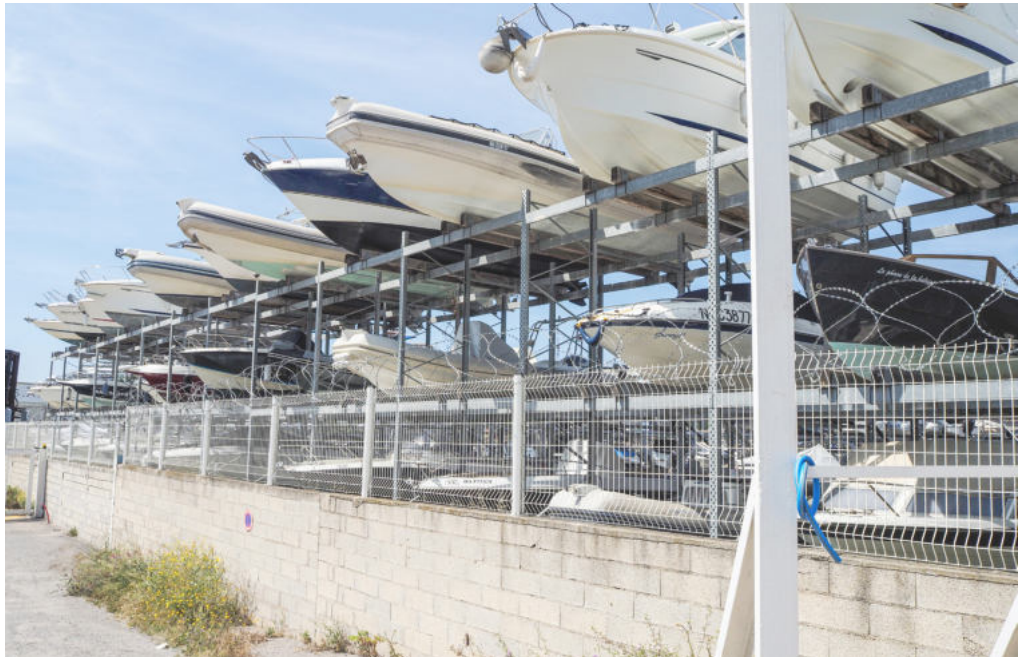
Fig. 137 - Boat storage sites in the Saumaty area, in the Rade Nord of Marseille (picture by the author, 2021).
