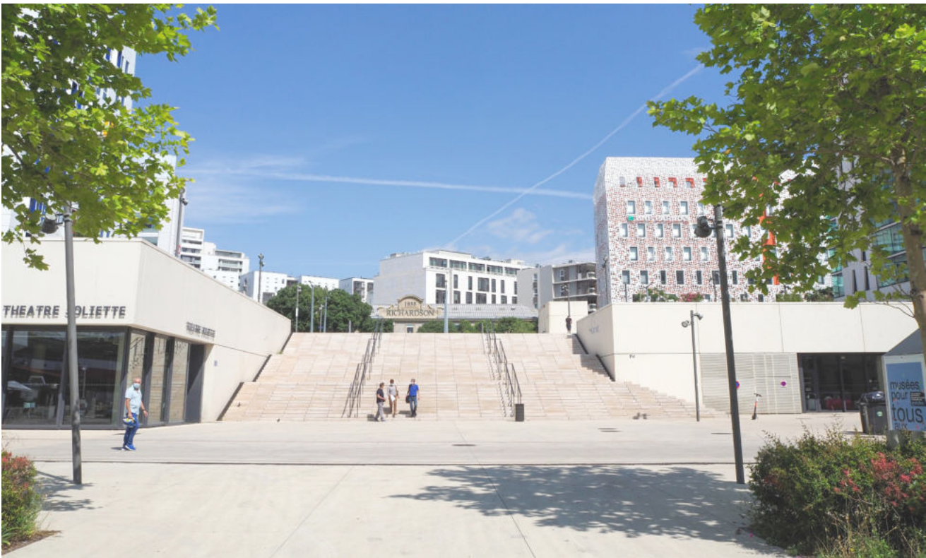
Fig. 46 - Place Henri Verneuil represents an important node of the Euroméditerranée district, as it connects various accommodation, cultural and administrative functions: however, it often appears not very frequented (picture by the author, 2022).
