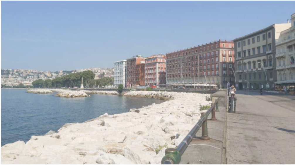
Fig. 115 - The promenade of the Mergellina area is one of the main walkway of the Neapolitan city, frequented by tourists and residents also for bathing purposes (picture by the author, 2022).
