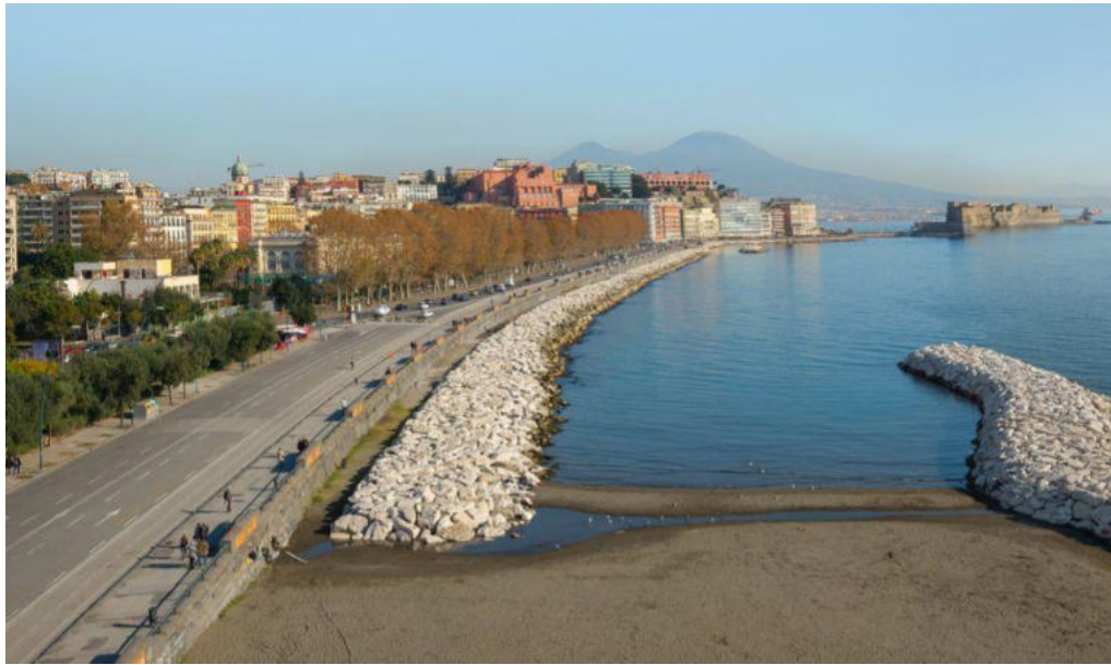
Fig. 132 - In Naples, the Riviera di Chiaia area is strongly characterized by the presence of artificial rocks parallel to the coast, designed as a defense against environmental risk but commonly used by Neapolitan users as a recreational space (source: V. De Bernardo, 2016).
