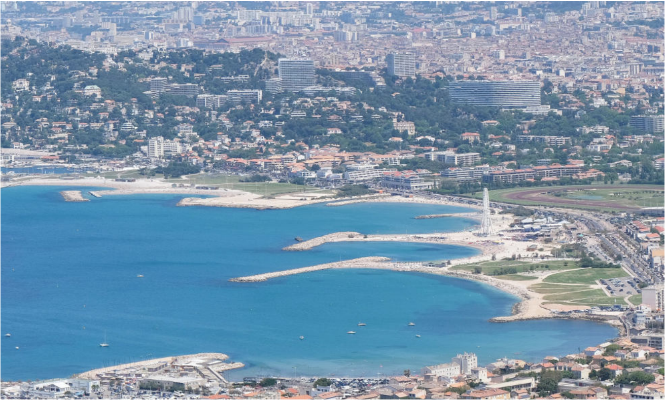
Fig. 44 - The wide Prado coastal park, with large open spaces for sports and bathing and commercial functions. Behind, the green area of Parc Borély (source: Hilader, 2019).
