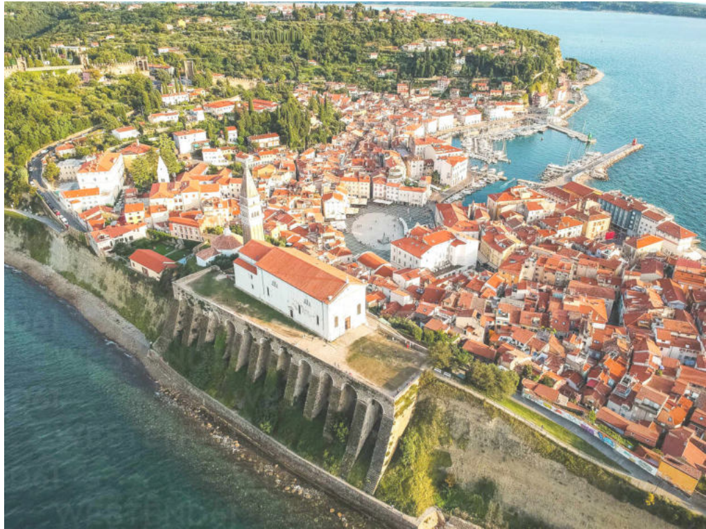
Fig. 7 - The land-sea interface includes urbanized and vegetated areas, for which an efficient planning and ecological balance is required. In the photo, the coastal interface of Piran, Slovenia (source: Amazing Aerial Agency).
