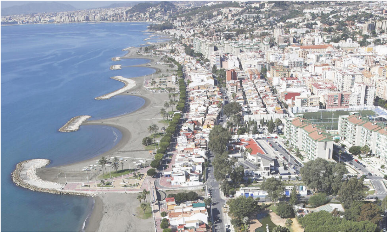
Fig. 60 - The pocket beaches system in the Pedralejo area, with its characteristic artificial reefs that help preserve the strips of coastal land used for bathing (source: J. Albinana, 2018).
