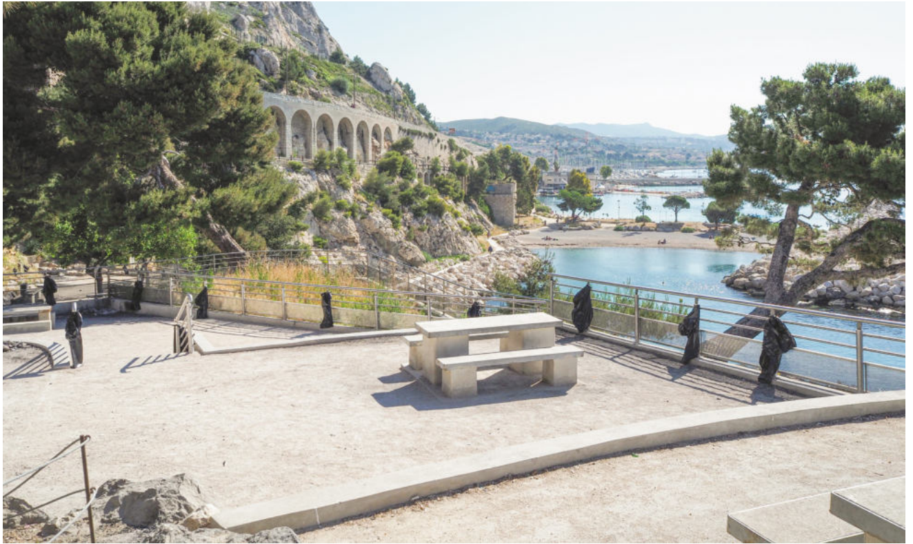
Fig. 52 - One of the accesses to the Corbières bathing system. In particular, the terraced steps within the public garden is shown: it is used as a social meeting place, although it is affected by a certain degree of neglect and denotes difficult accessibility (picture by the author, 2021).
