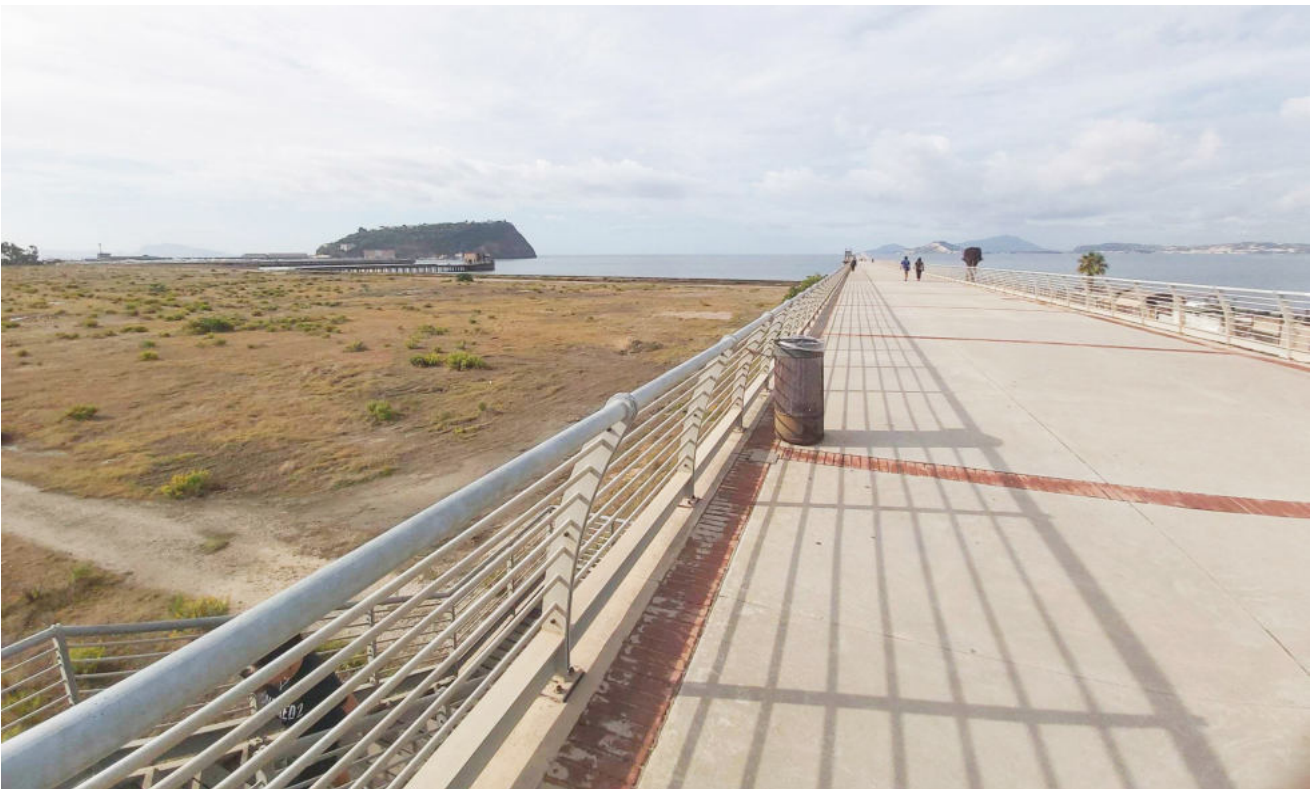
Fig. 67 - The long pedestrian walkway of the Bagnoli pier, frequented at different times of the day for recreational, social and sporting functions, represents a landmark in the Neapolitan city-sea interface (picture by the author, 2021).
