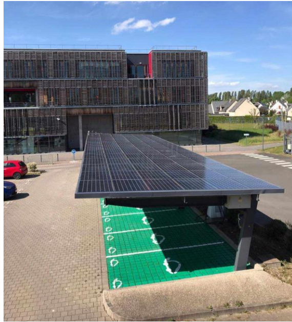
Figure 106: PV-powered charging station installation for nine spots.
