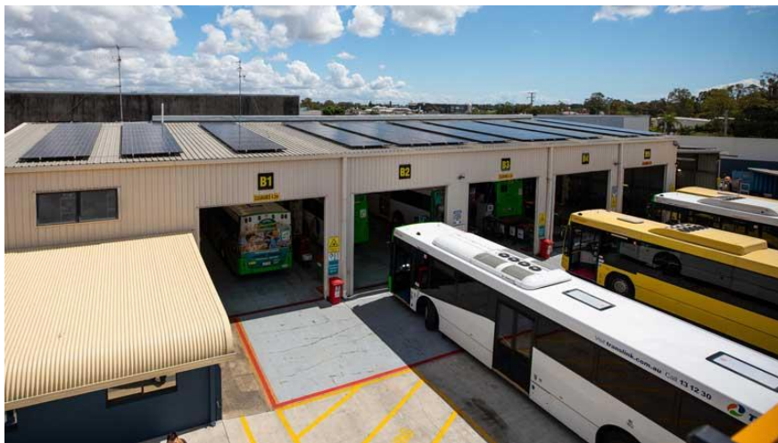
Figure 20: Transdev electric bus PV-powered depot [36].
