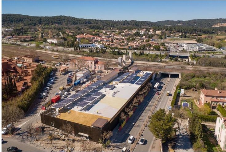
Figure 19: PV-powered infrastructure at Gardanne's train station [35].
