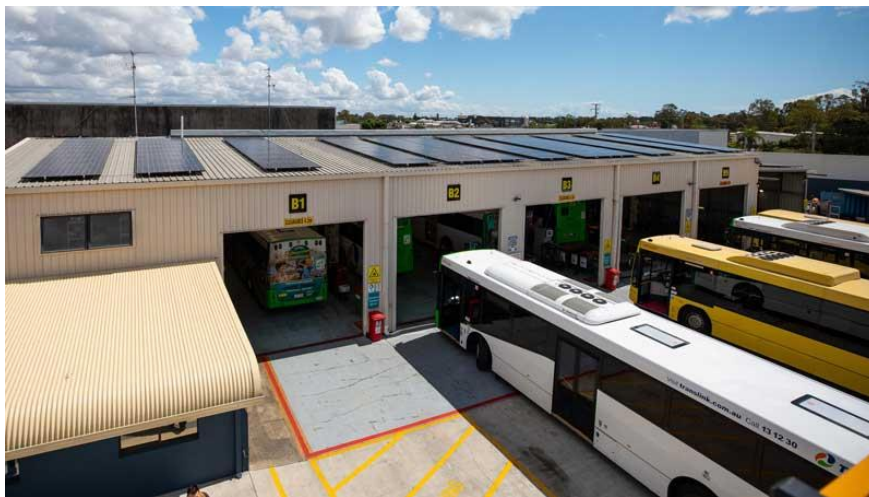
Figure 20: Transdev electric bus PV-powered depot [36].
