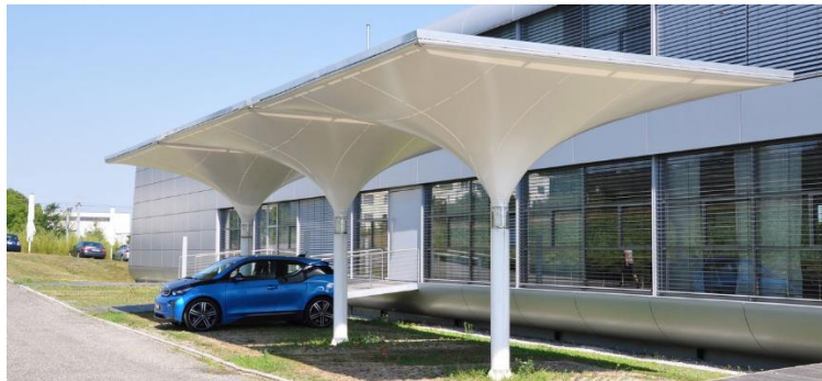
Figure 17: MDT-tex Solar Carport [32].
