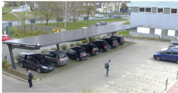
Figure 34: PV parking shade installation for nine spots.
