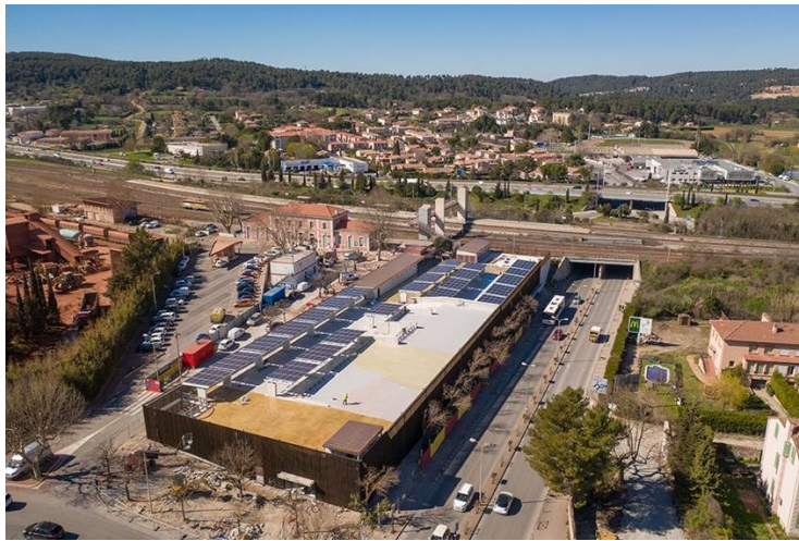
Figure 19: PV-powered infrastructure at Gardanne's train station [35].
