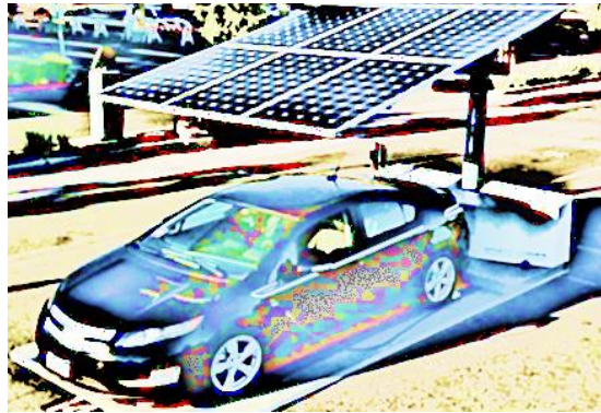
Figure 27: PV parking shade.
