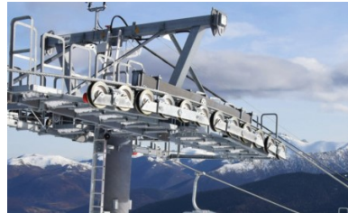
(b) Support roller battery - TSF4 Bisorne / Ax-les-Thermes
