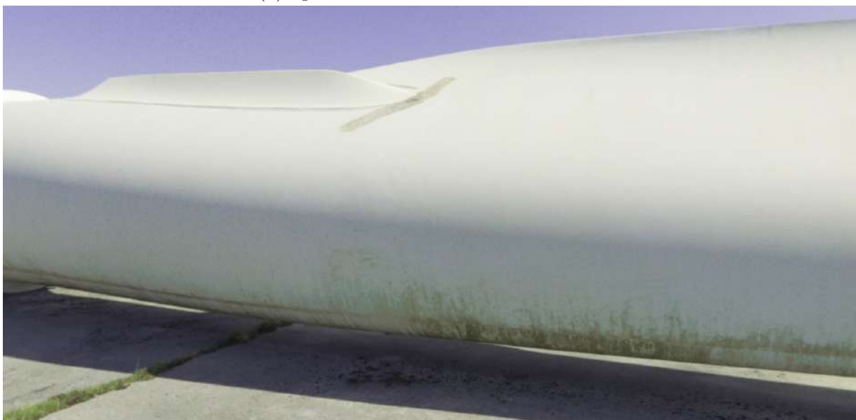
(b) Repair patch near the spoiler location
