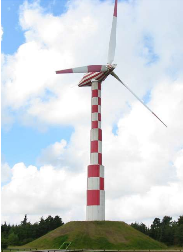
Figure 1.8 – First multi MegaWatt turbine (2MW) build by teachers and students from Tvind school in 1978.
