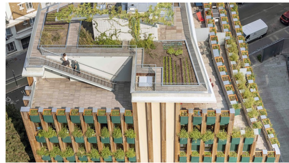
Figure 37: Edison Lite - Paris 13e ©Manuelle Gautrand Architecture
