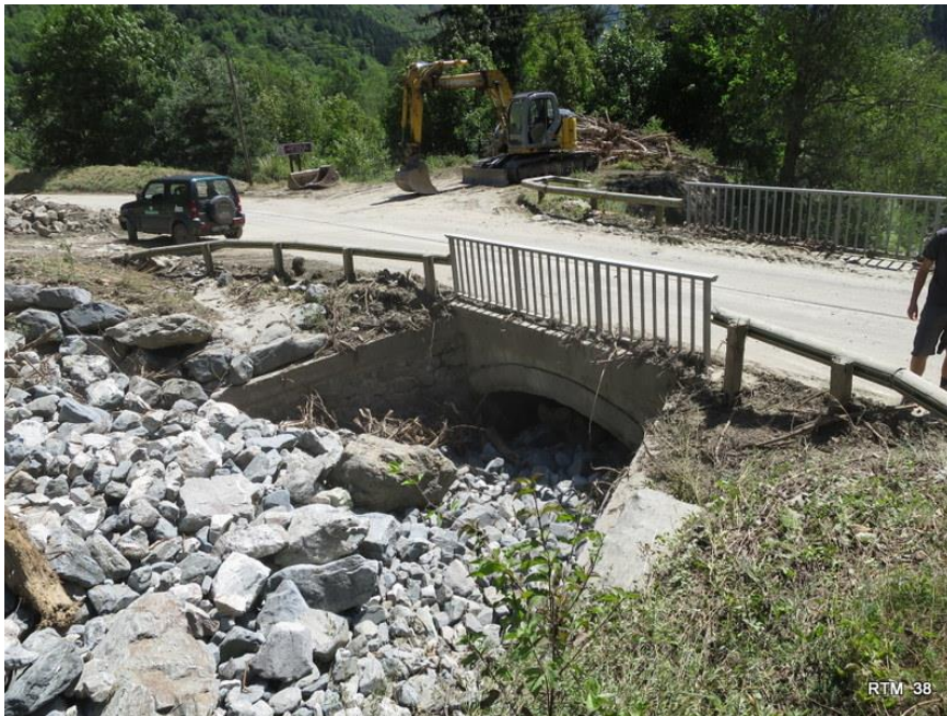
Figure 2.2 : Effect of a sediment pulse at a bridge section of the Ruisseau de la Gorge (France), a stream that was known by local engineers as having been inactive for decades. The transported material was much finer ( D_{50} = 96 \text{ mm} , D_{84} = 169 \text{ mm} ) than the bed in place ( D_{50} = 250 \text{ mm} , D_{84} = 413 \text{ mm} ).
