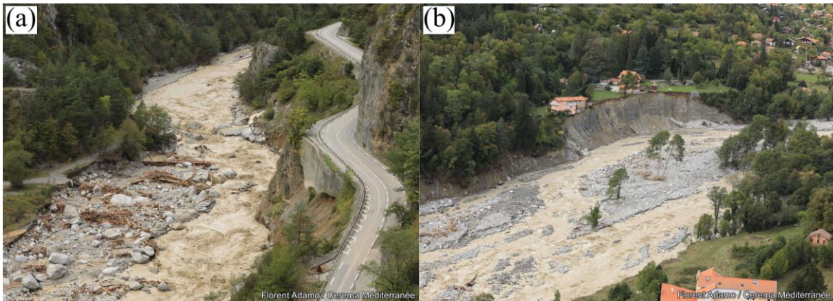
Figure 1.7 : The impact of extreme floods. In October 2020, the Maritime Alps were hit by the Storm Alex that caused dramatic floods in several mountain catchments. The event was associated with very high water discharges and intense sediment transport that disrupted large parts of the fluvial landscape. (a) Bank erosion and deposition of material on roads. (b) Large bank collapse next to the Saint-Martin-Vésubie village and strong impact on river morphology. Photo credits: Florent Adamo/Cerema.
