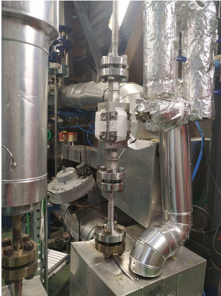
Figure 7.20: DIOGEN test section implemented on BIKINI installation.
