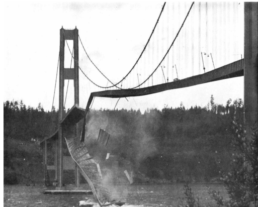
FIGURE 1.2: Collapse of Tacoma bridge due to flutter instabilities [8].
