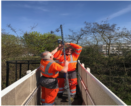
(a) Road manager operators installing material
