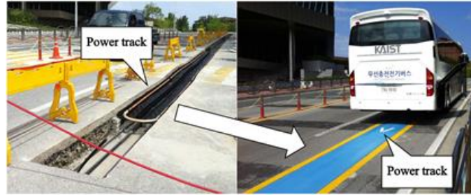
Figure 1.16 KAIST OLEV: dynamic wireless charging EVs with a large transmitter [33]
