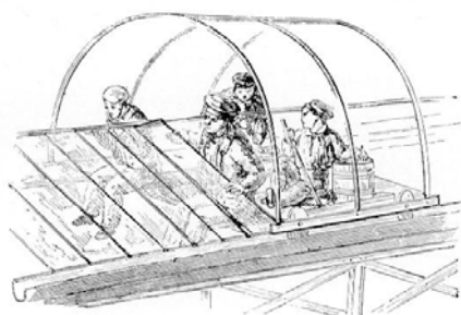
36. Paxton's ingenious glazing waggon, which could be covered over in weather and which ran on wheels, carrying the glazing crew their equipment.
