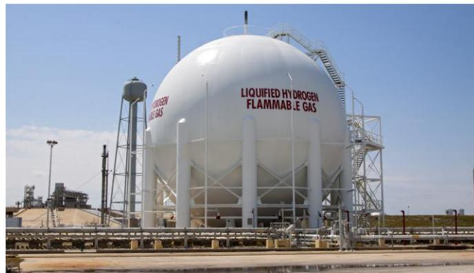
*Figure 2.11. Example of liquid hydrogen tank for space applications (NASA, 2015)*
