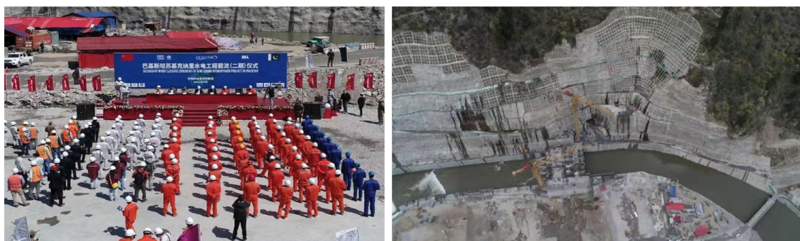
Figure 2.33: Construction work on Suki Kinari HPP (Source: CPEC AUTHORITY (25-04-2022))
