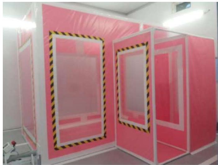
Figure 5-2 Picture of the real airlock with its flexible vinyl walls
