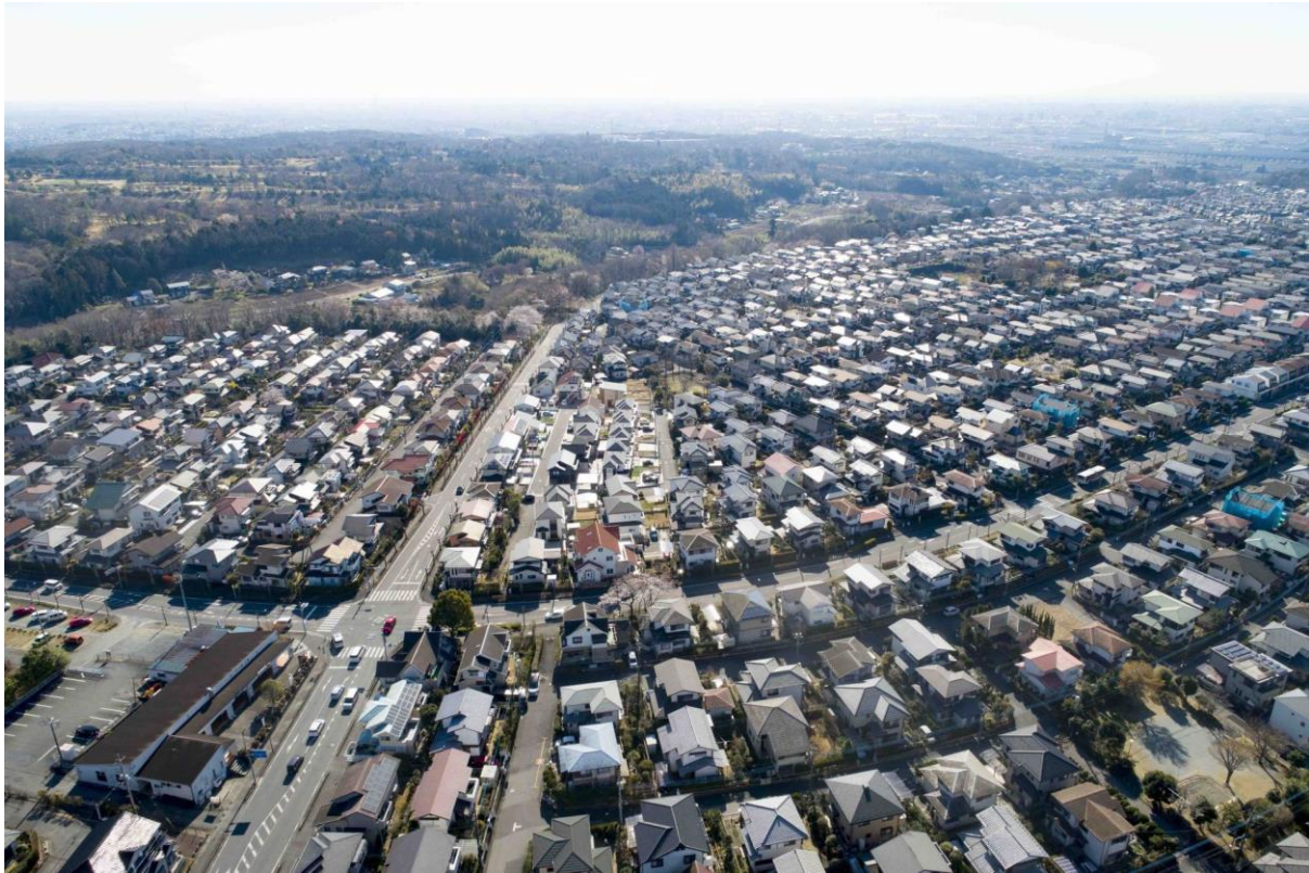
Fig.1.30. A view of the Kamikatsu Urban Ecovillage
