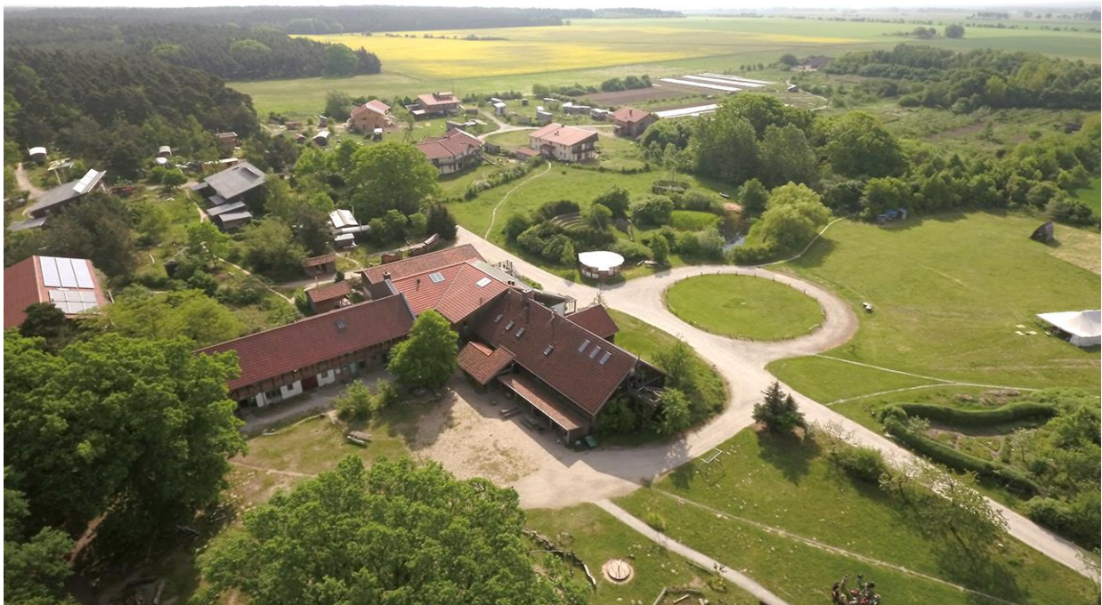
Fig.1.14. Sieben Linden Ecovillage: landscape view
