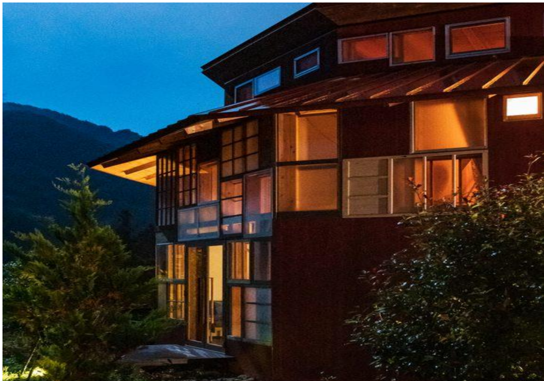
Fig.1.29. Co-Housing in Kamikatsu Urban Ecovillage
