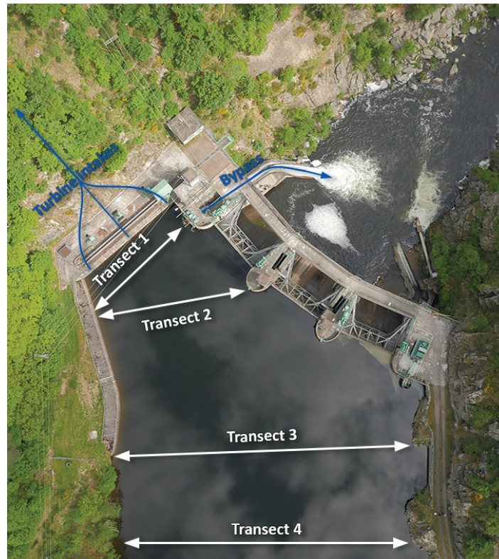
FIGURE 3.3 – View of Poutès dam and field measurement locations (with ADCP transects).
