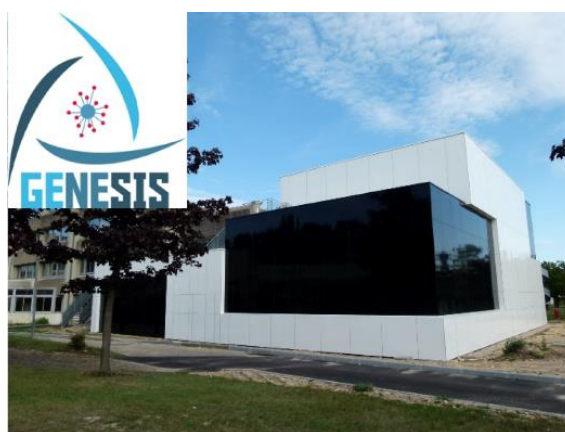
Figure 175: The GENESIS platform building at GPM.
