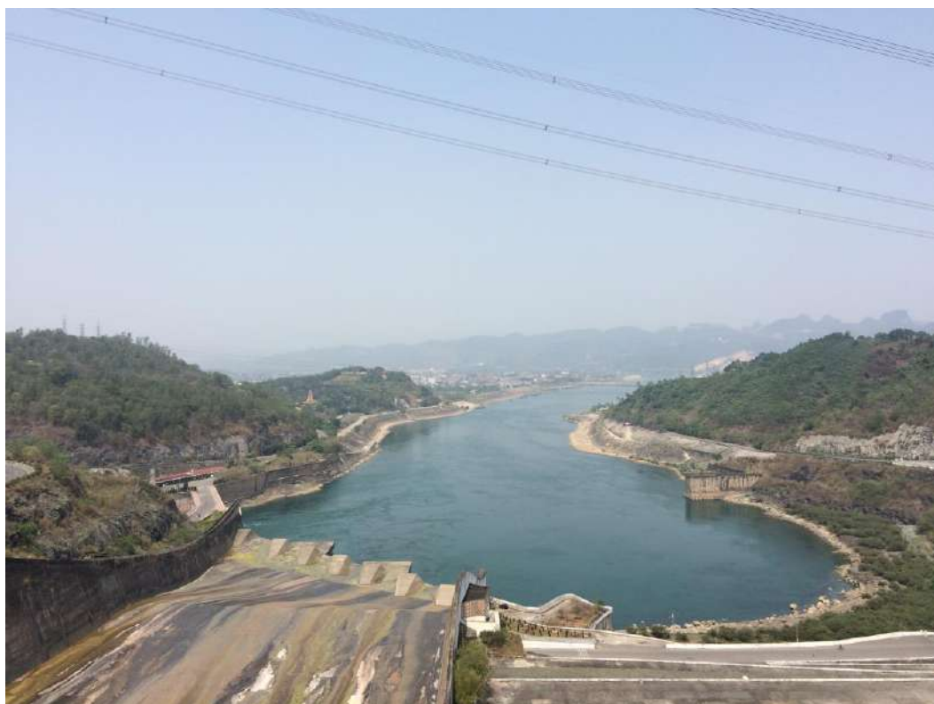
Figure 2-8 The downstream of the Hoa Binh dam.
