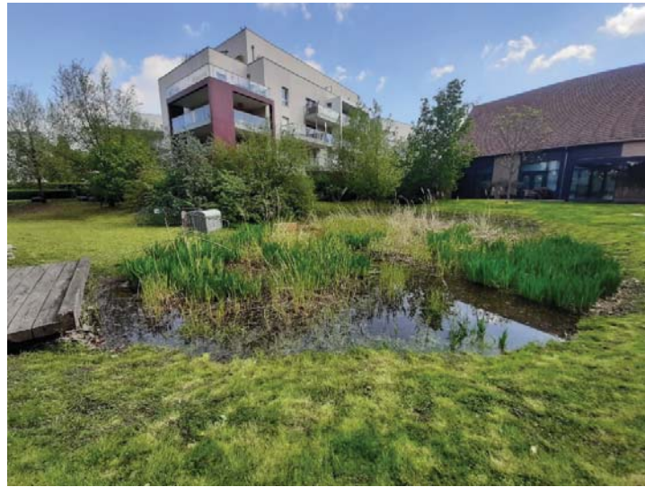
Figure E 1. Infiltration pond in spring 2021.
