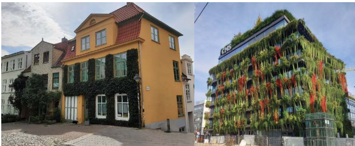
Figure 9. 4. Vegetated facades (Lübeck, Germany) with an earth-bound system (left) and system-bound at the CMS building (Calwer-Passage, Stuttgart, Germany) (right) (Pictures: Tobias Junginger, Marie Hundhausen).
