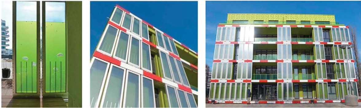
Figure 9. 3. The Bio-Intelligent Quotient house in Hamburg with algae bioreactors (Elrayies, 2018). Bioreactors are used for biomass generation.
