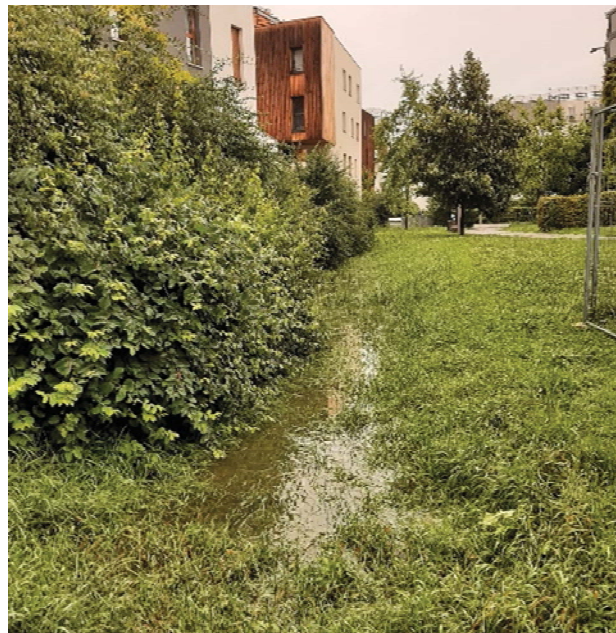
Figure E 2. Infiltration trench in summer 2021.
